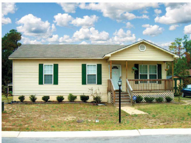
Closed crawlspaces represent both a new business opportunity and a risk management tool for many different stakeholders in the construction industry.
