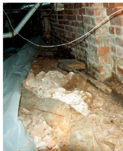
A more typical vented crawlspace in North Carolina exhibits a poor quality vapor retarder, if any, and various complications such as debris and clutter.
