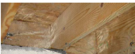
This floor-insulated crawlspace has a termite inspection gap at the top of the vapor retarder. Note that penetrations are thoroughly sealed with mastic.
